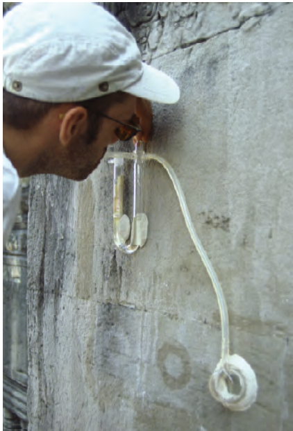
Figure 10: Tests of air permeability help to determine the success of the removal.
