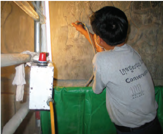
Figure 8: Thick salt layers have to be thinned out before they are reduced by water poultices.
