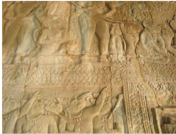
Figure 17: Joints after closing with adapted mortar.
