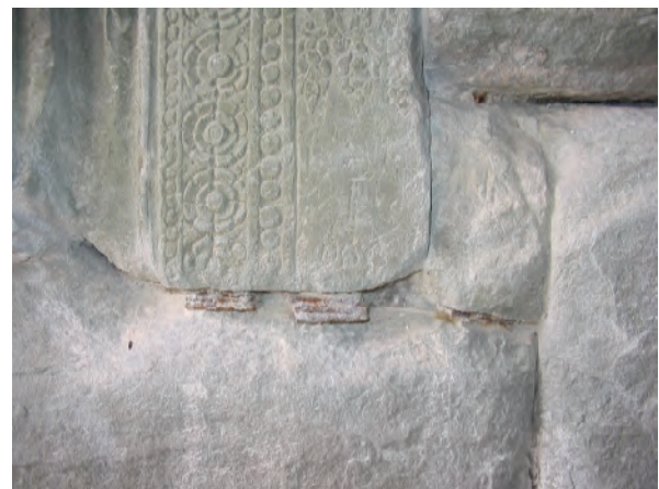
Figure 7: Rusting iron jacks from former restoration affect the original stone by bursting.
