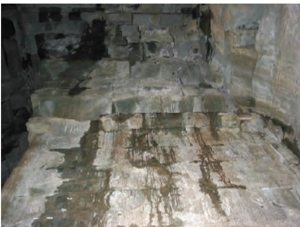
Figure 6: Water infiltration from open joints and leaking roofs is a very serious damaging factor.
