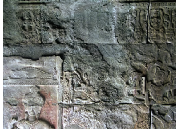
Figure 5: Thin scales are a common damage feature in the Southwest Pavilion.
