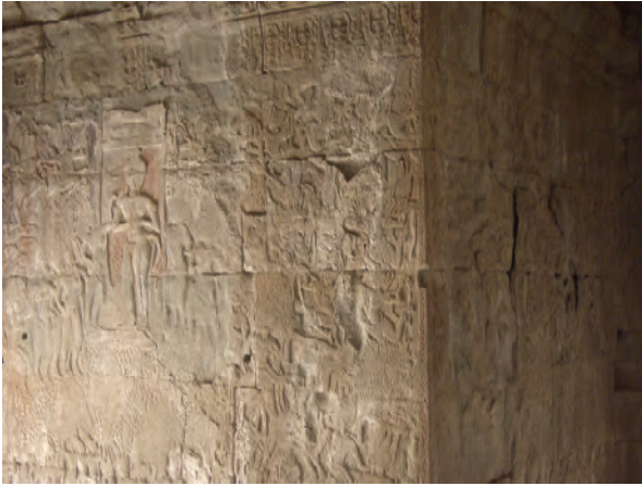
Figure 4: Thick scales are typical decay phenomena with the Angkor Vat sandstone.
